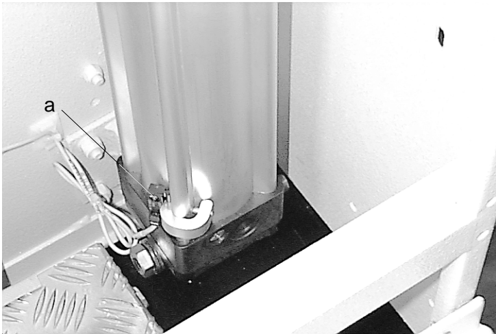
Fig F.7: Pillar 2, below a Limit switch roof brush up
